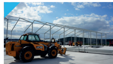
Frames are manufactured to BS6399 / BSEN1991 for wind & snow loads.
